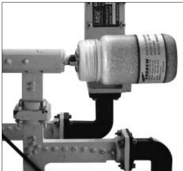
Static Desiccator SD-002A attached to 2 Port Combiner of 4.5 m ESA.
