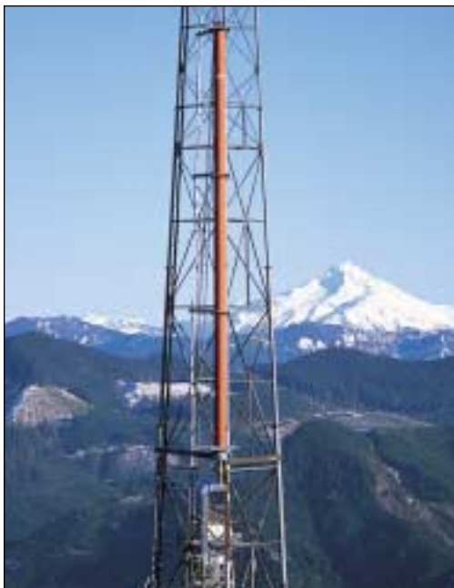
KWBP Channel 32/31, Salem, Oregon The side-mounted, dual adjacent, TRASAR antenna operates both NTSC & DTV signals simultaneously.
