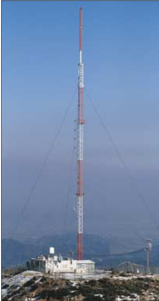
TRASAR® V-Series antenna KNTV for channel 11 features pressurizable radome to withstand salt air coastal environment.
